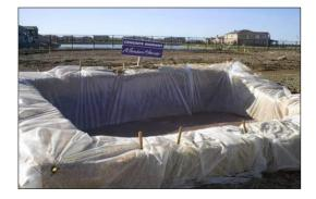
Plate 4-3 Concrete washout area
