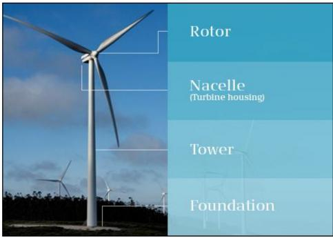
Plate 4-1 Wind turbine components
