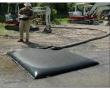
Plate 4-6 Silt Bag with water being pumped through
