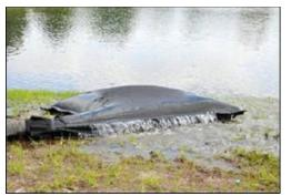
Plate 4-7 Silt bag under inspection
