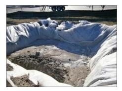
Plate 4-4 Concrete washout area
